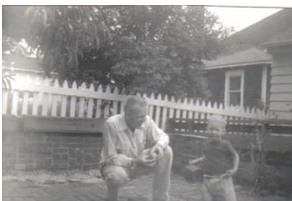
Ben built a brick sandbox next to the brick wall behind him in this picture.
